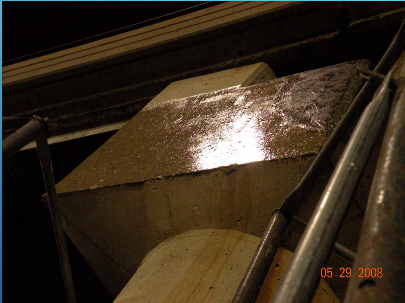
Application of Primer Material on Pier 1 Surface
