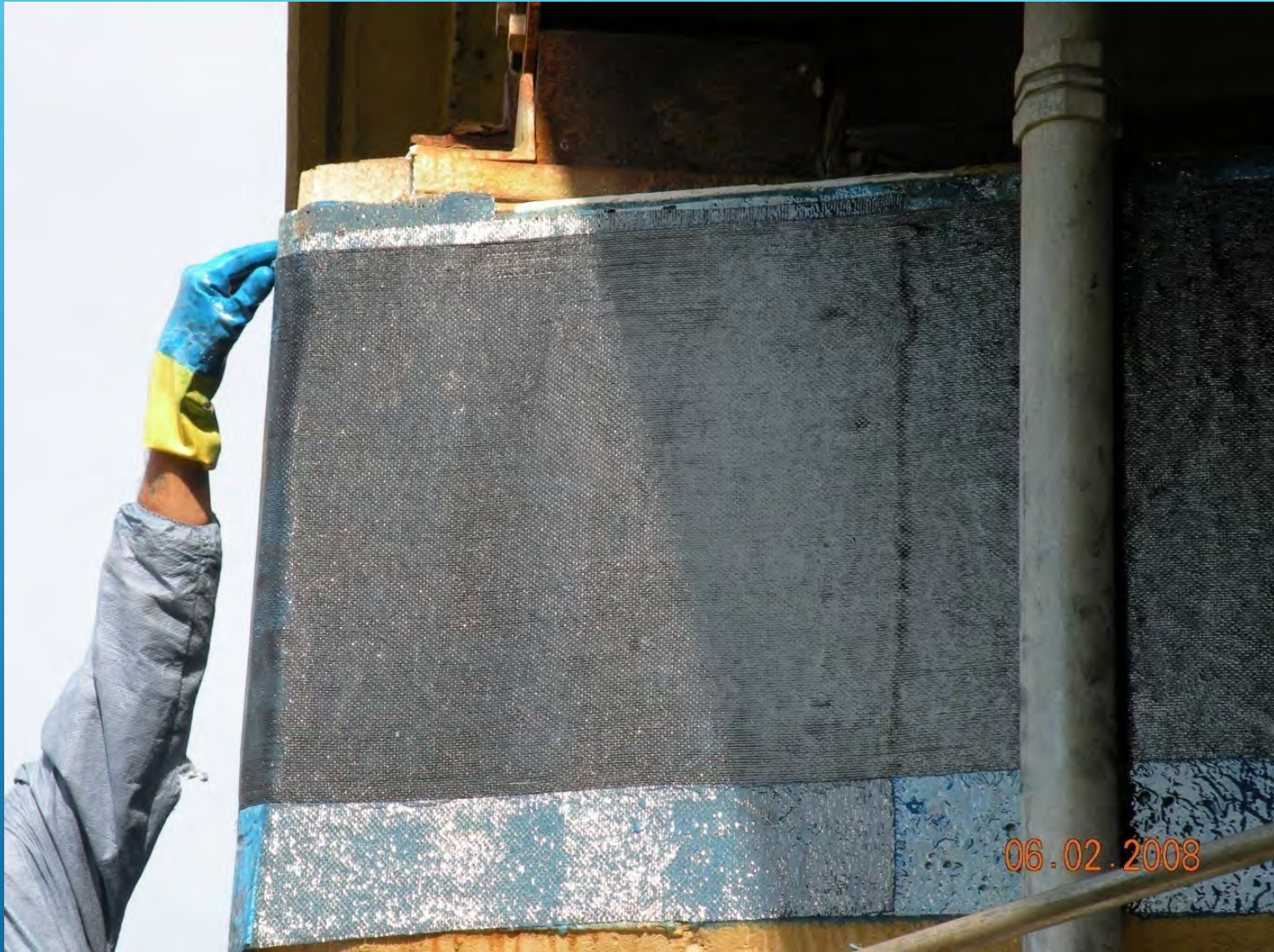
Application of First Horizontal Layer of CFRP on Pier 1
